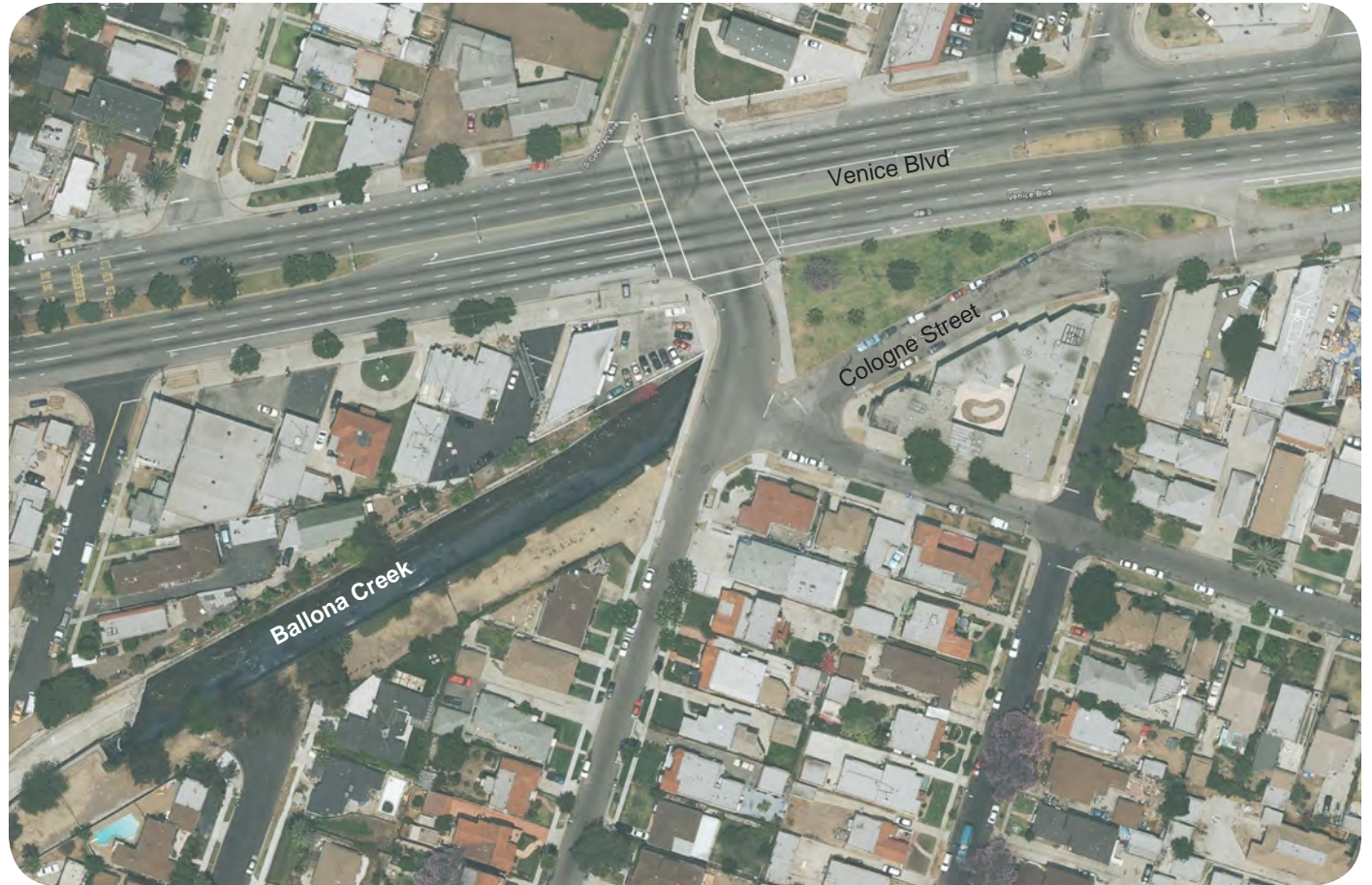
Existing Conditions: Aerial Photograph
