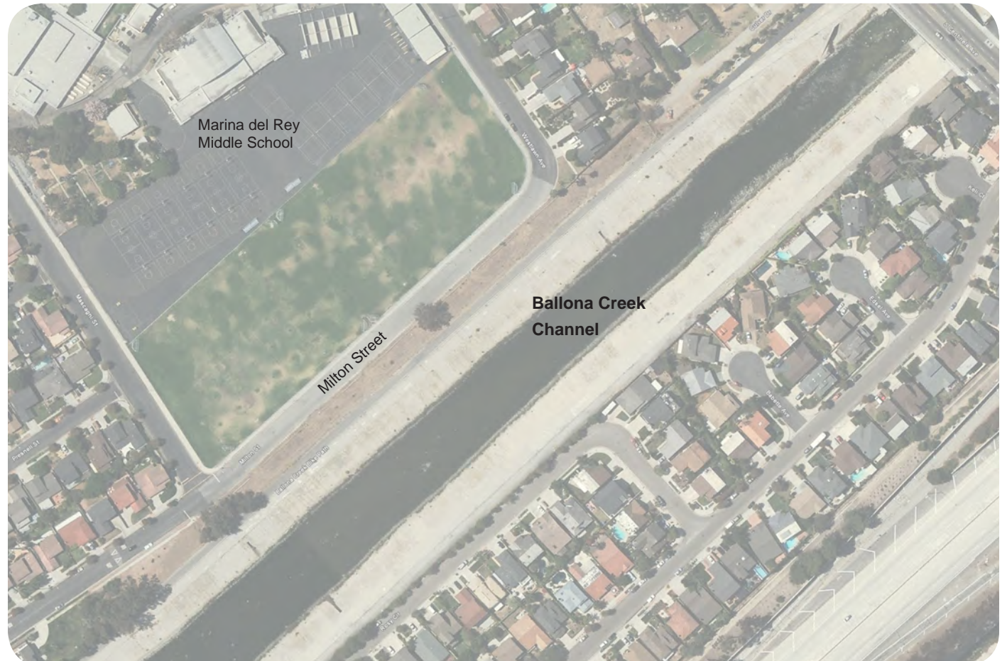
Existing Conditions: Aerial Photograph
