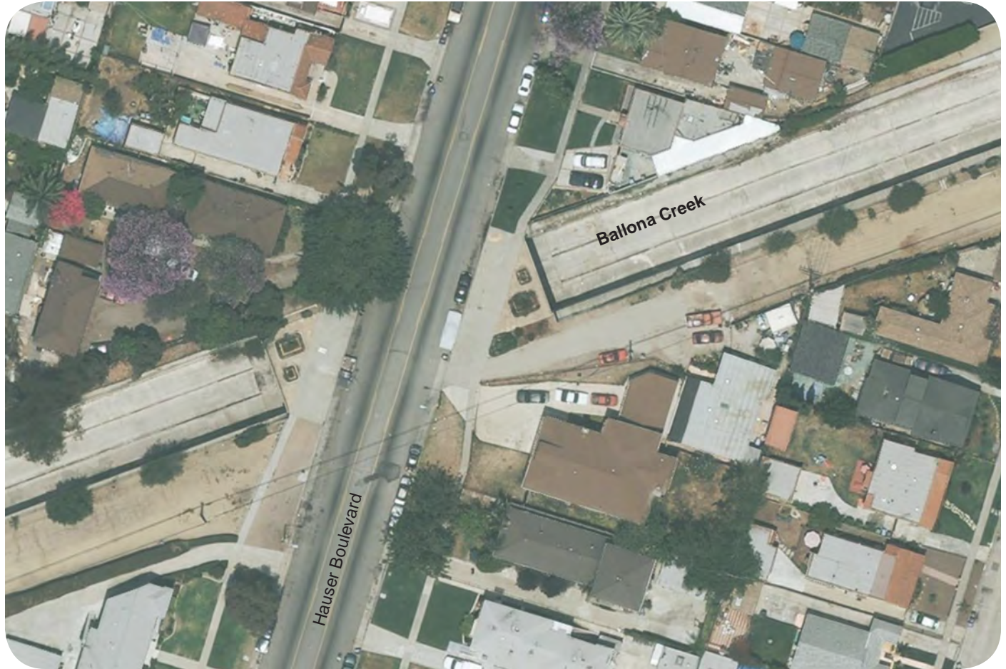
Existing Conditions: Aerial Photograph
