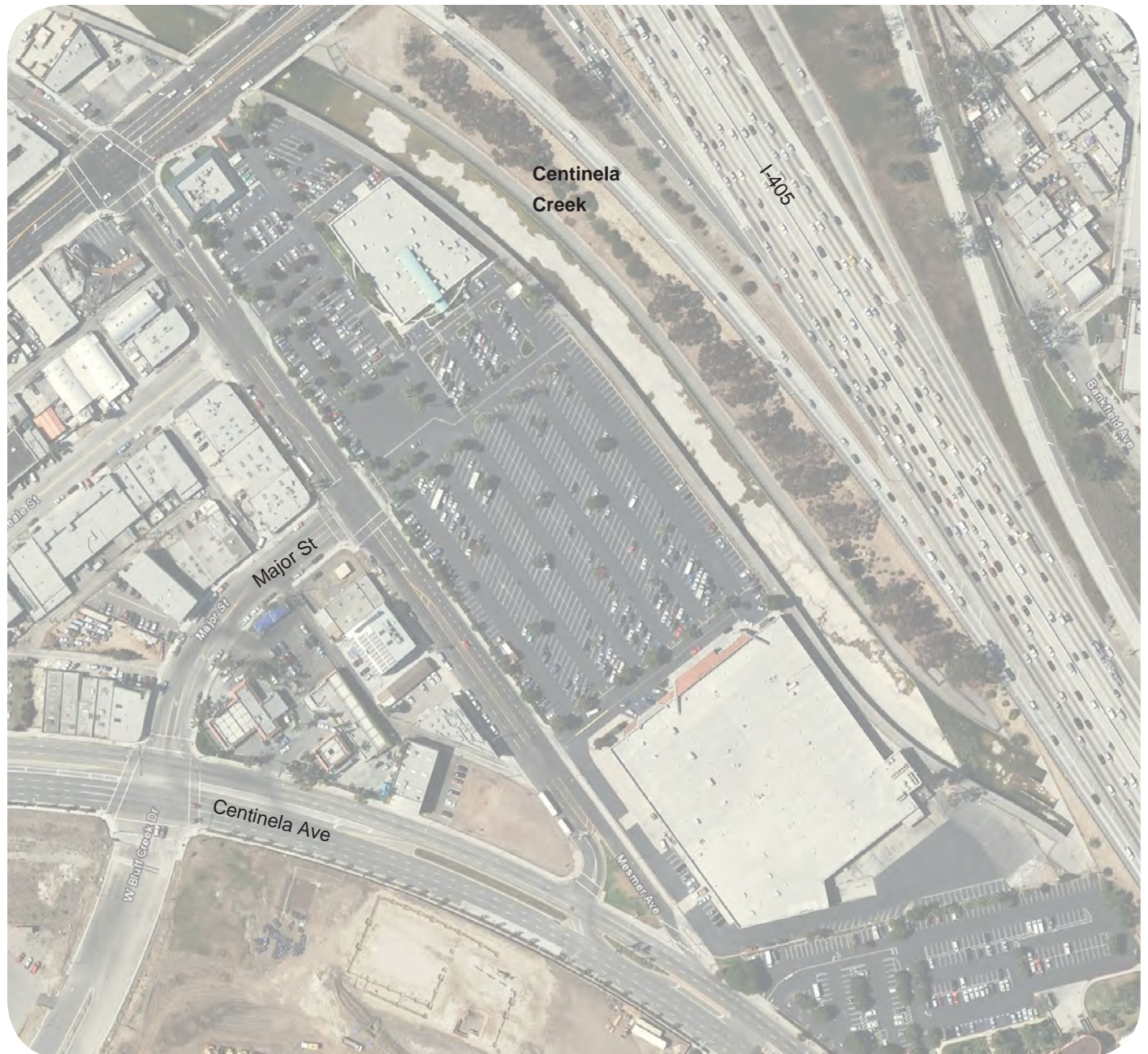
Existing Conditions: Aerial Photograph
