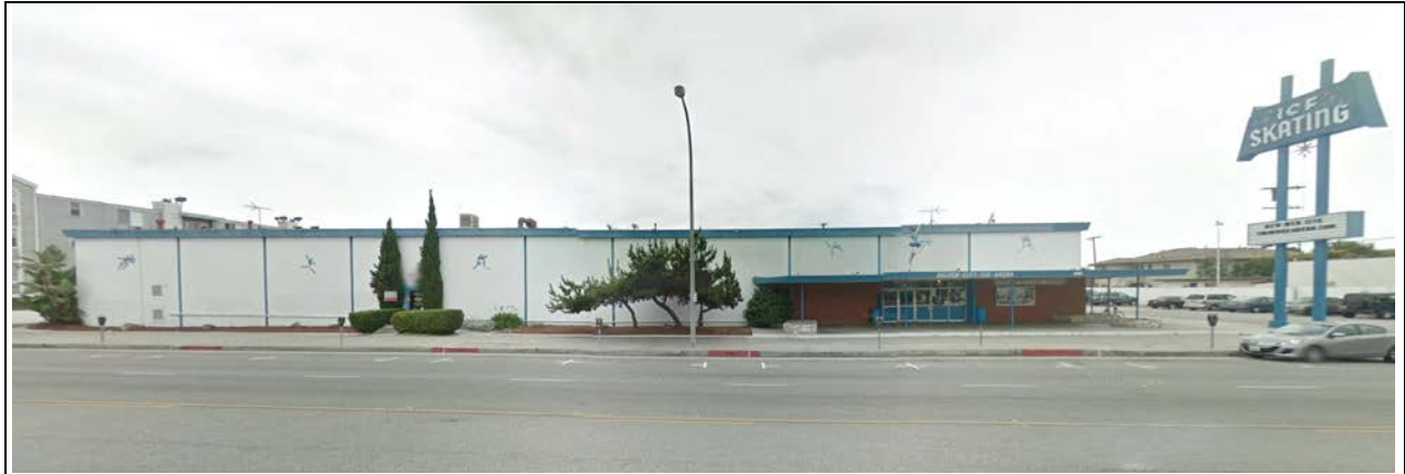
View west of east (main) façade and signage. Google Street View, accessed March 2014.
