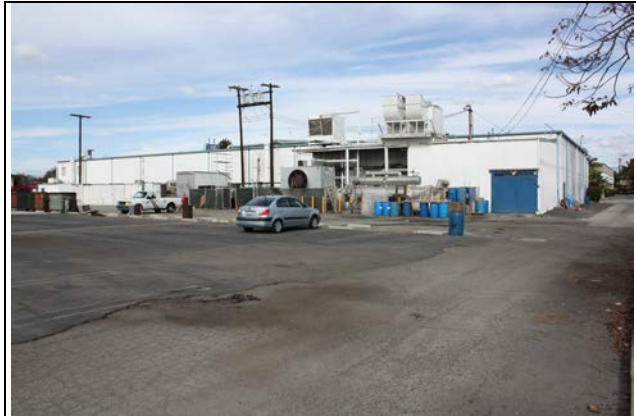
Utility area at south end of the rear of the building. ARG, 1/31/14.
