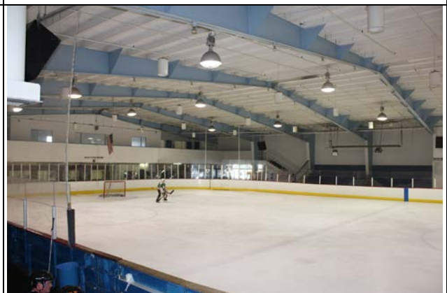
View northeast of rink with mezzanine and gallery at north end. ARG, 1/31/14.
