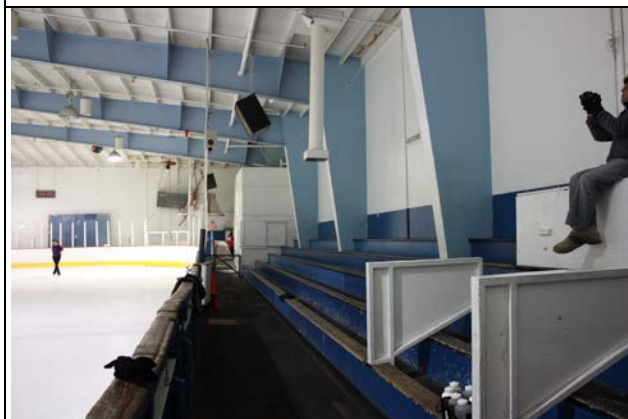
Steel trusses and spectator seating on west side of rink, view south. ARG, 1/31/14.
