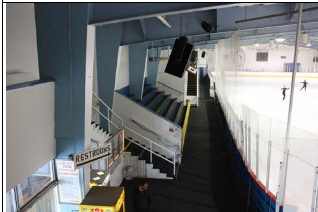
Steel trusses and spectator seating on east side of rink, view south. ARG, 1/31/14.
