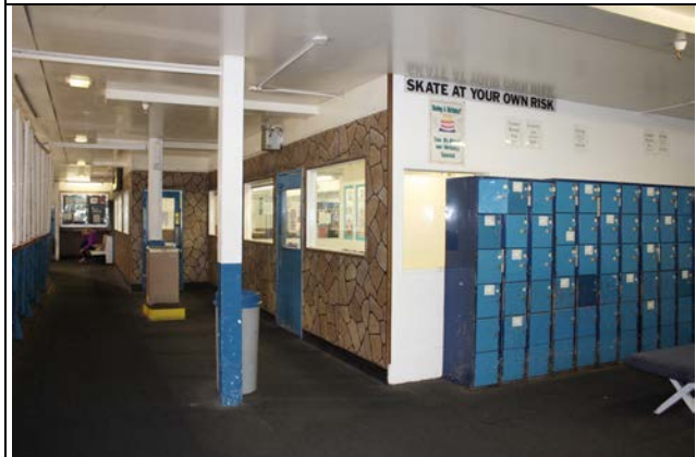
View northwest of locker area (foreground, right) and enclosed changing room. ARG, 1/31/14.
