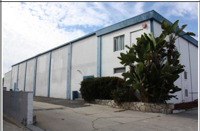
View northwest of south façade with planters at corner. ARG, 1/31/14.
