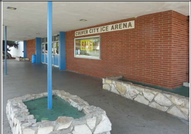
View southwest within entrance porch. ARG, 1/31/14.
