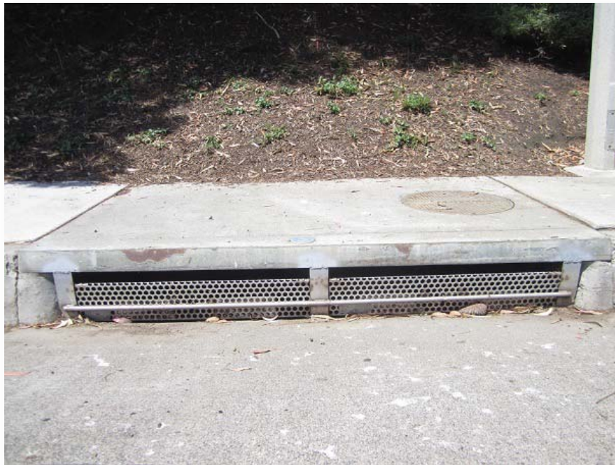
Automatic Retractable Screen (ARS) Across Curb Opening
