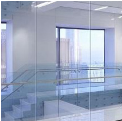
SSG BUTT JOINT STOREFRONT SYSTEM
