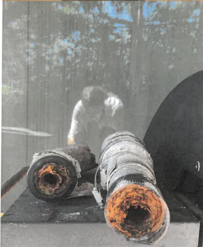
Old Sewer Pipe
