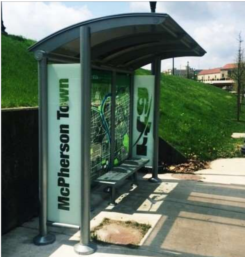
Below: Aluminum arch cantilever roof with partial side walls, custom ceramic frit walls.
