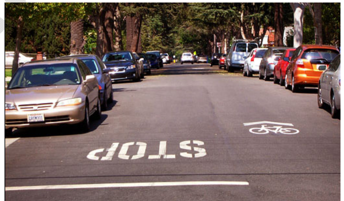
Bicycle route with sharrows on Irving Place, Culver City
