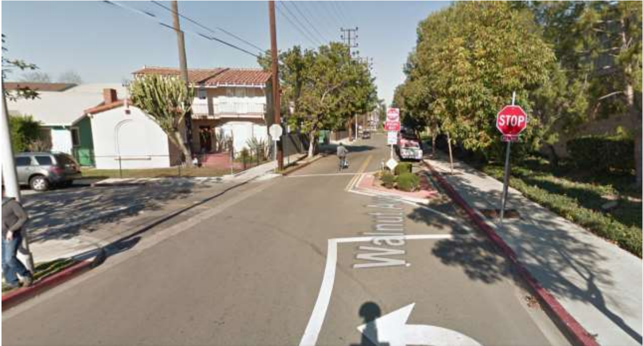
Figure 11. Channelization at Walnut Avenue and Elm Street Intersection.
