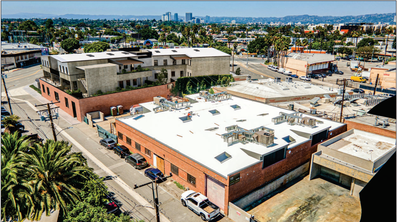
Oblique view of the project looking northwest
