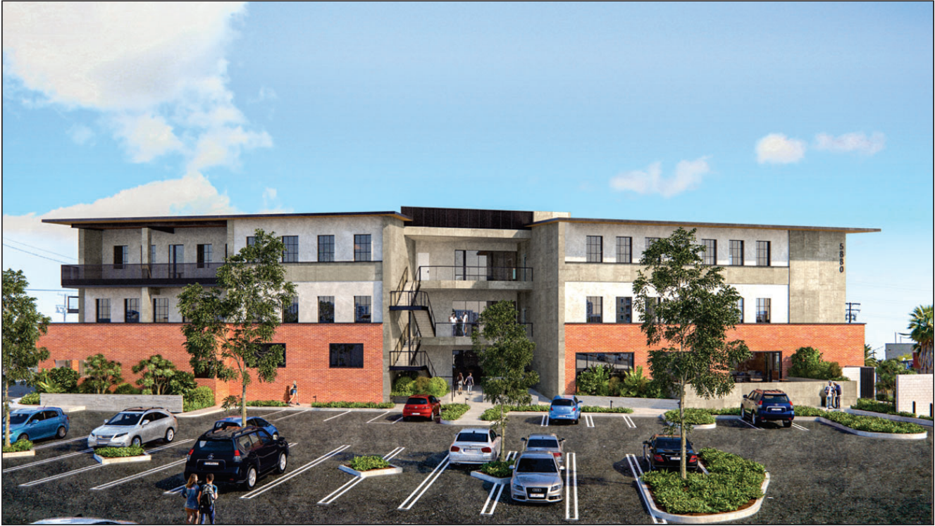
View of west entrance
