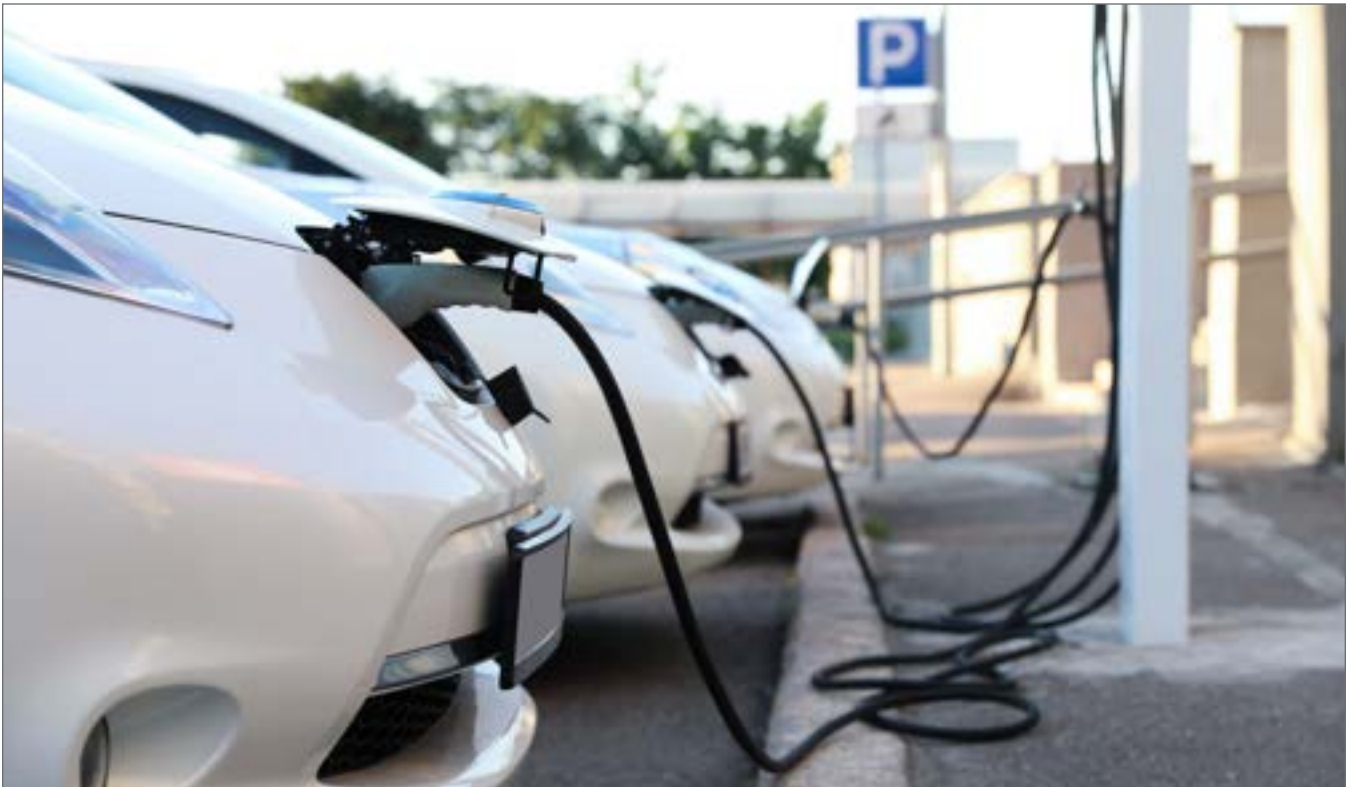
Electric vehicle charging
