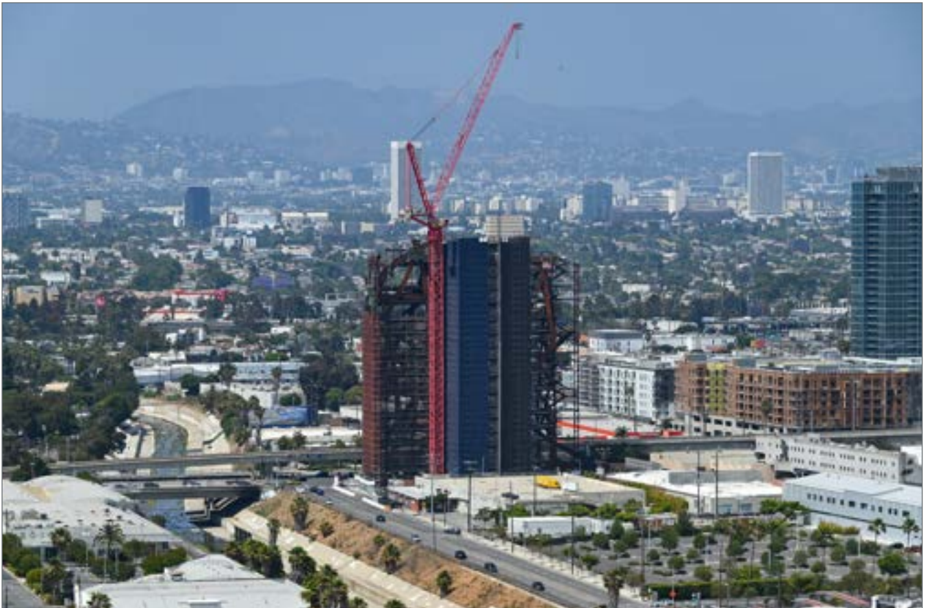
New construction near Culver City
