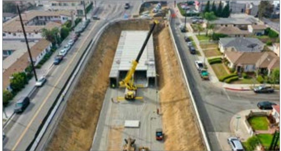
Construction of Culver Blvd stormwater infrastructure. Source: Michael Baker Intl.
