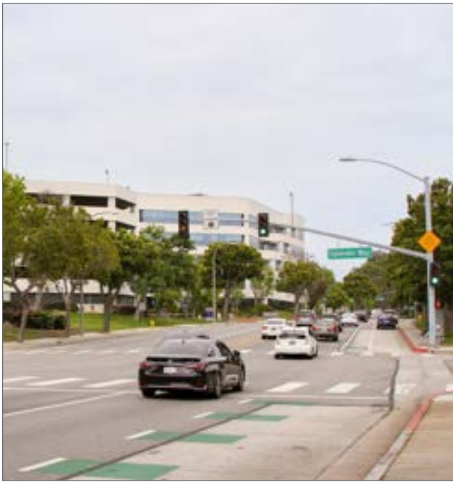
Primary arterial in Culver City
